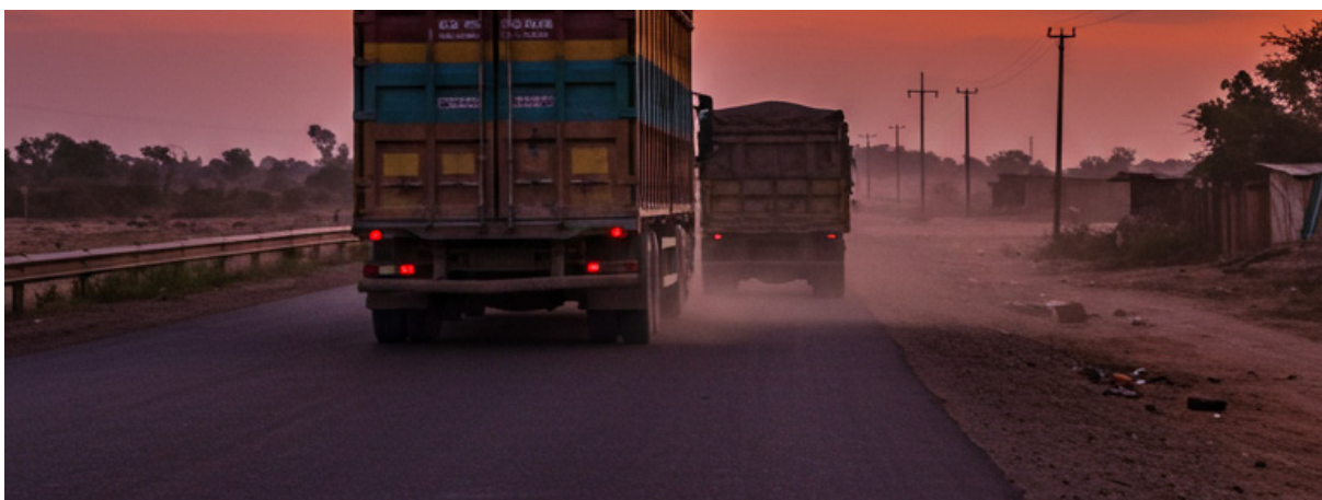
A single carriageway reflecting the current state of most ECOWAS road corridors
