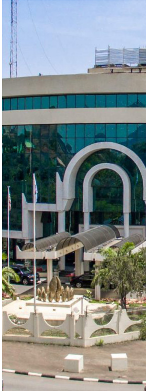
ECOWAS Commission Headquarters in Abuja, Nigeria
